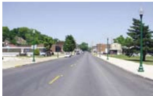
Decorative Street Lights
