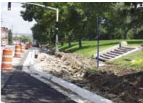
Curb Improvement to St. John Avenue
