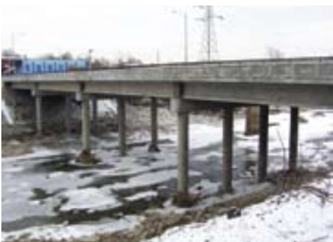
Broadway Bridge over River Des Peres
