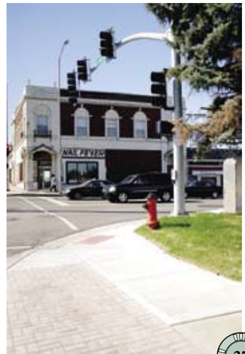
75th & Troost Street Improvements
