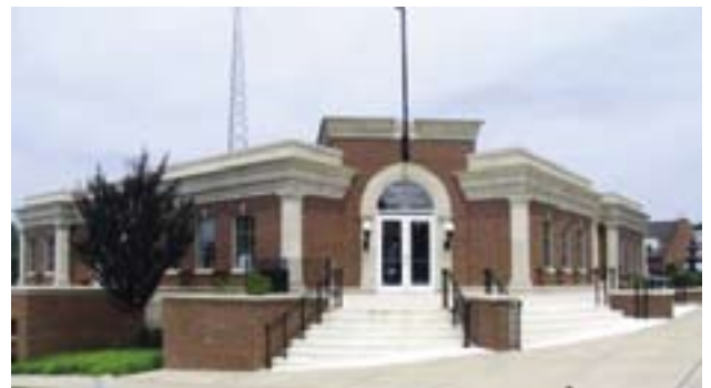
New Police Station
